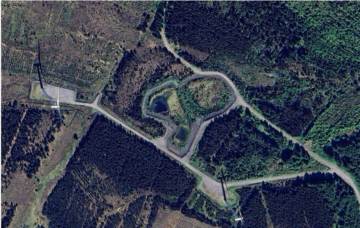
Photo 3 – Recent aerial photo of the backfilled borrow pit cells on the Garvagh Glebe Wind Farm
