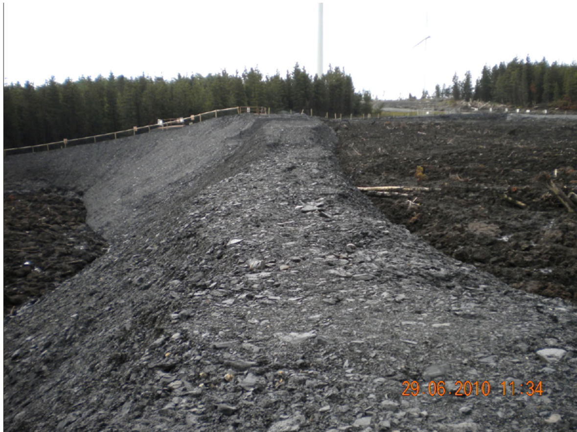
Photo 2 – Backfilled borrow pit cells on the Garvagh Glebe Wind Farm, Co. Leitrim
