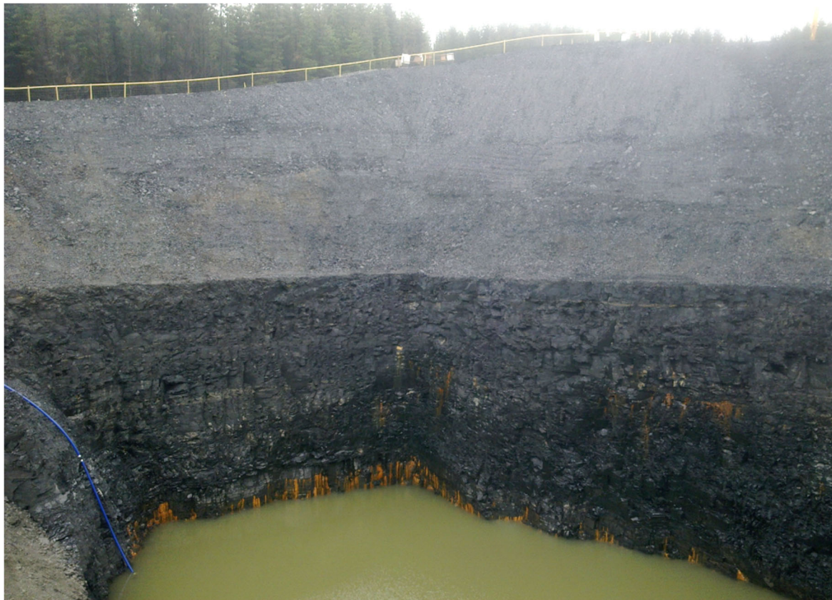
Photo 1 – Fully developed borrow pit cell prior to backfilling on the Garvagh Glebe Wind Farm
